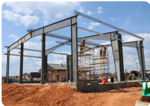
Pre- Engineered Building Shed
